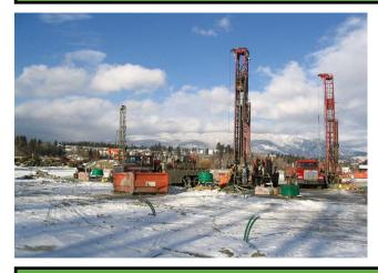
Vertical boreholes of the GeoExchange field go down to depths of 500 ft (~150 m).
